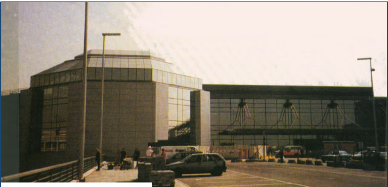
Exterior view of new terminal building.
